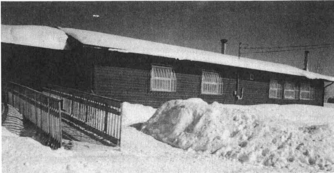
Marten Falls Nursing Station
